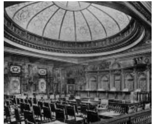
ABOVE, LEFT: Rambusch design drawing for three-armed wall sconce based upon photographic and period research. RIGHT: Courthouse building and central chamber as they appeared in the early 1900s.
